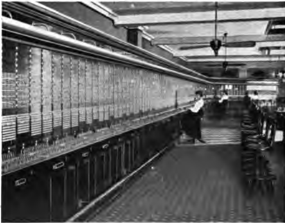
General View Central Battery Board
